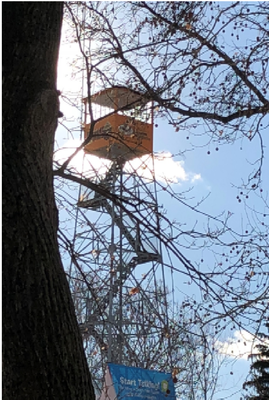
Armintrout Fire Tower at Ohio Natural Resources Park, Ohio State Fairgrounds, Columbus, Ohio (January 2018)
