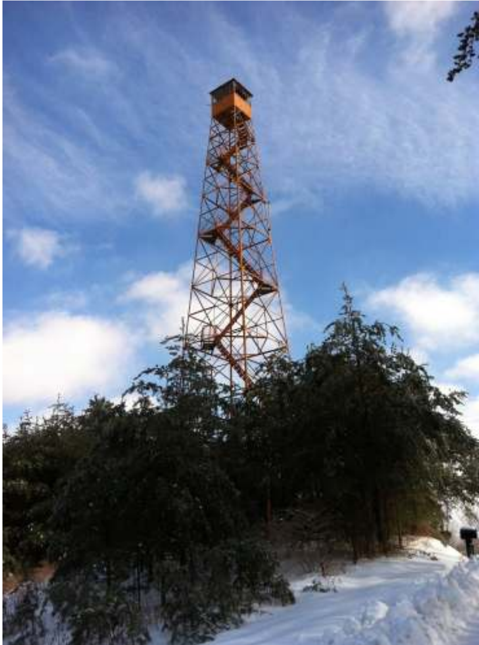
Rockbridge (Sugar Grove) Fire Tower at its original site on Firetower Rd, Berne Township, Fairfield County Ohio. To be relocated to Charles F. Alley Memorial Park, Berne Township, Fairfield County, Ohio A City of Lancaster, Ohio Parks and Recreation Department facility. (2015)
