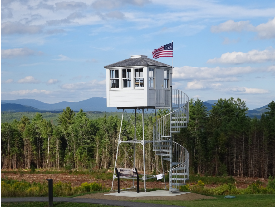
The finished product - The former Squaw Mountain fire tower is now erected at the Greenville visitor center.
