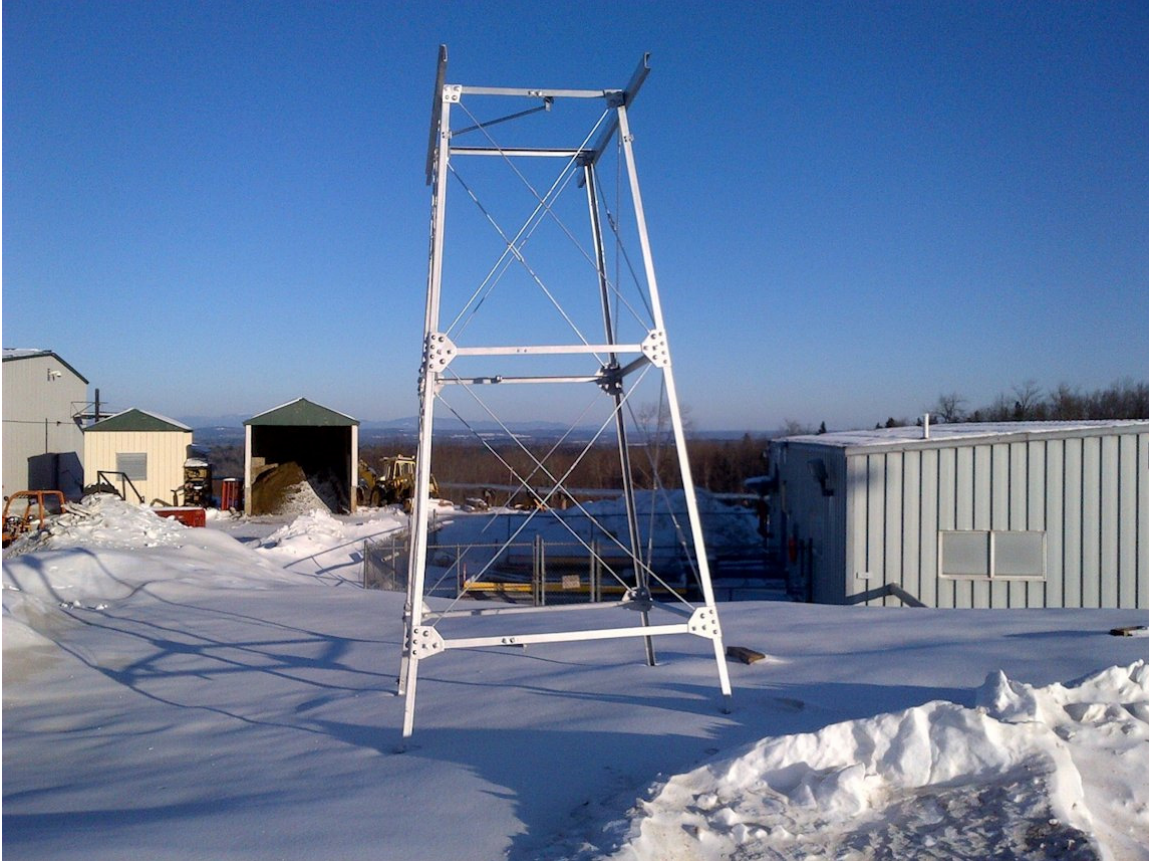
The 1919 Big Moose Tower after restoration in January 2015.
